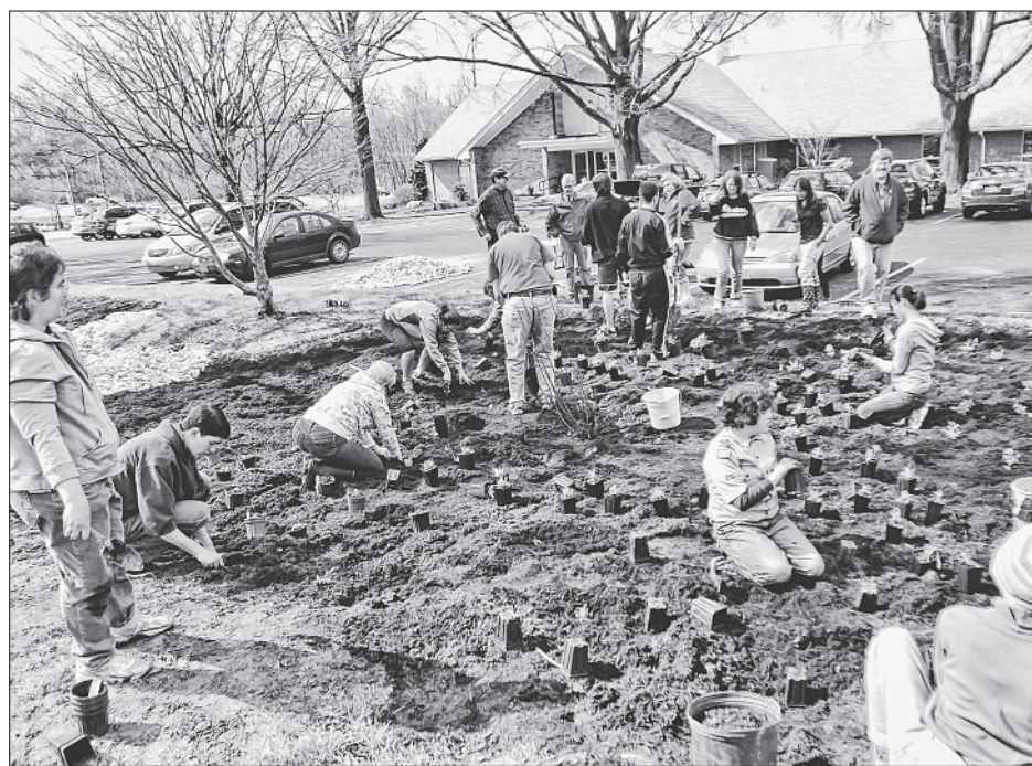
Volunteers convened at Limestone Presbyterian Church on Saturday to plant a rain garden that will filter chemicals that run off the parking lot when it rains.
